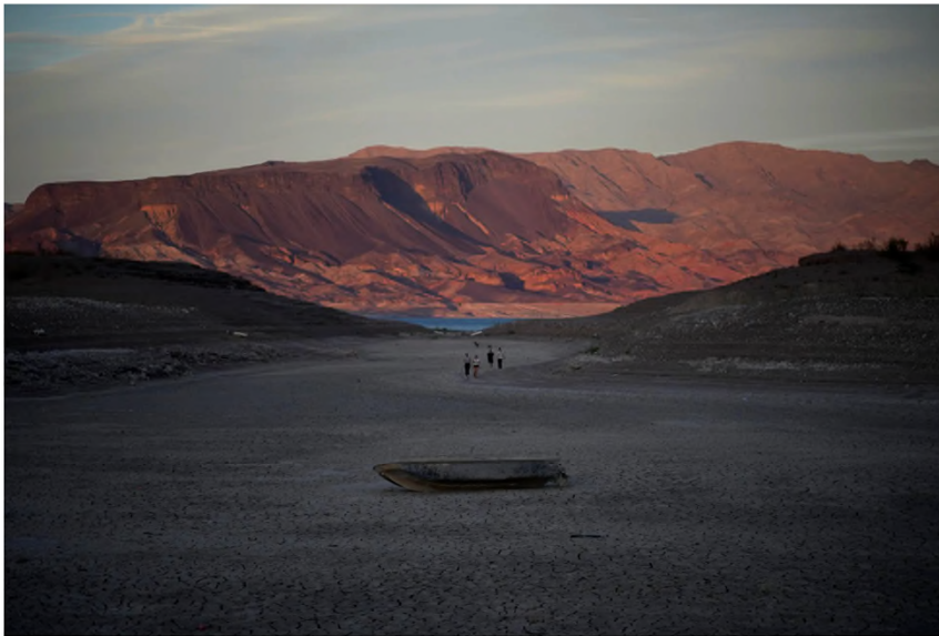
Lake Powell: Powers the Glen Canyon Dam Generation Station
